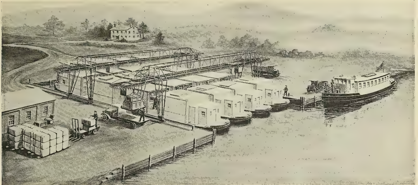
Fig. 4.—Proposed Barge Terminal, Showing Use of Gantry Cranes for Transferring Freight from Barges to Automobile Trucks
